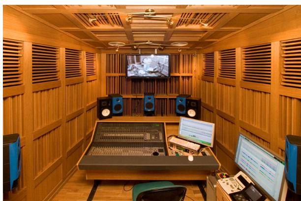
Fig. 6. – RES Media Studio, designed by MyRoom principles. Side diffusers are air transparent, order  $N=13$ . Behind front speakers is fractal diffuser of order  $N=7$  and  $M=7$ , it is air transparent too.
